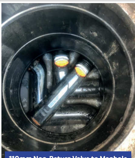
110mm Non-Return Valve to Manhole
