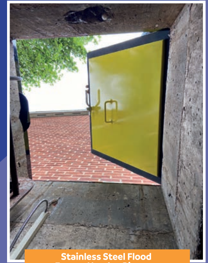
Stainless Steel Flood Escape Hatch - Bicester
