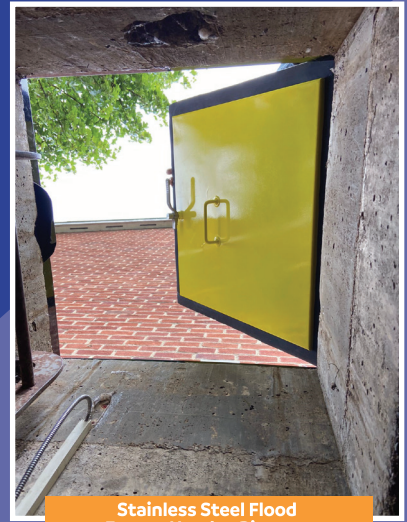
Stainless Steel Flood Escape Hatch – Bicester
