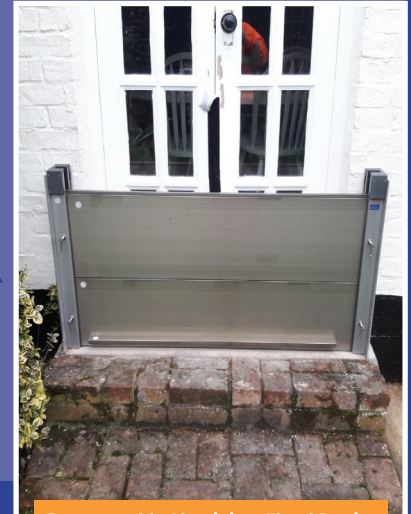
Demountable Aluminium Flood Barrier
