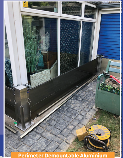
Perimeter Demountable Aluminium Flood Barrier to Conservatory
