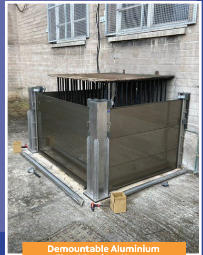
Demountable Aluminium Flood Barrier - Newry
