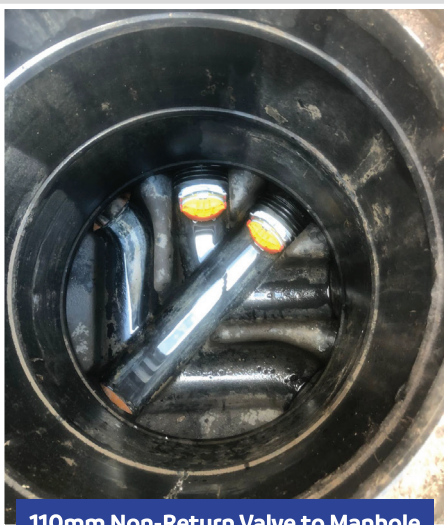
110mm Non-Return Valve to Manhole
