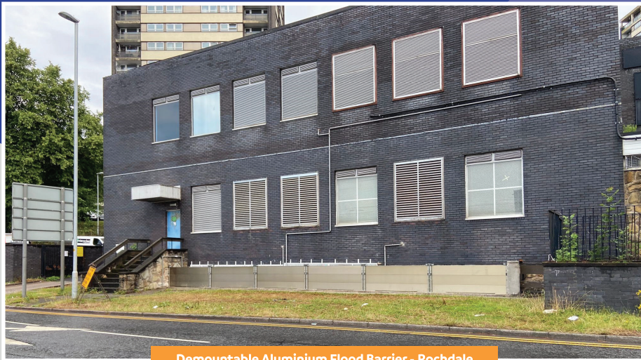
Demountable Aluminium Flood Barrier - Rochdale
