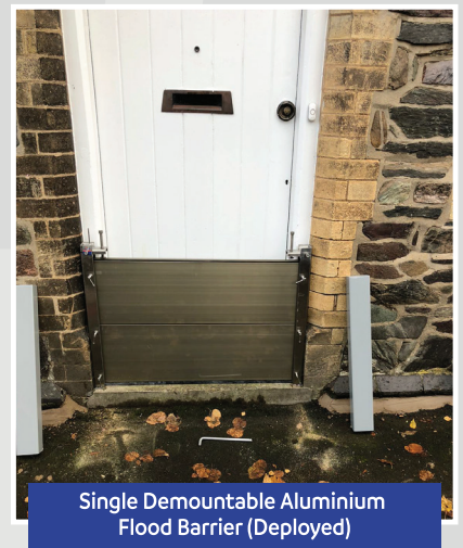
Grade II Listed Property - Demountable Aluminium Flood Barrier
