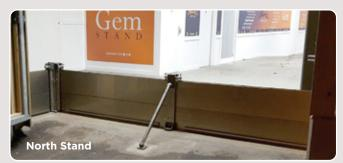
The Lakeside Flood Barrier was selected as the preferred protection method due to its user-friendly nature and quick deployment method.
