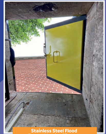
Stainless Steel Flood Escape Hatch - Bicester
