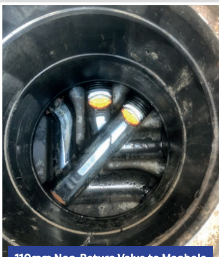
110mm Non-Return Valve to Manhole
