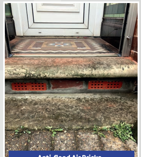
Anti-flood Air Bricks
