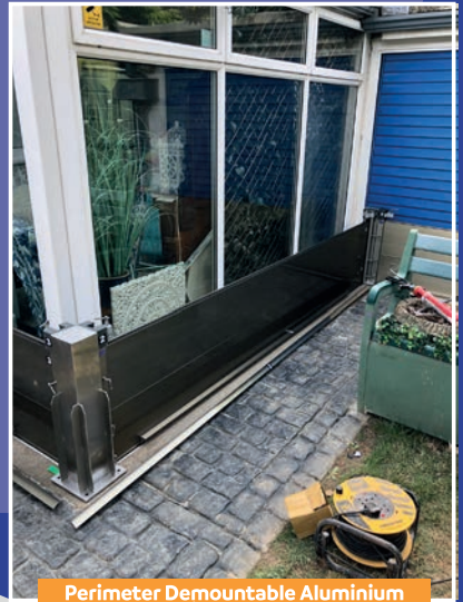
Perimeter Demountable Aluminium Flood Barrier to Conservatory
