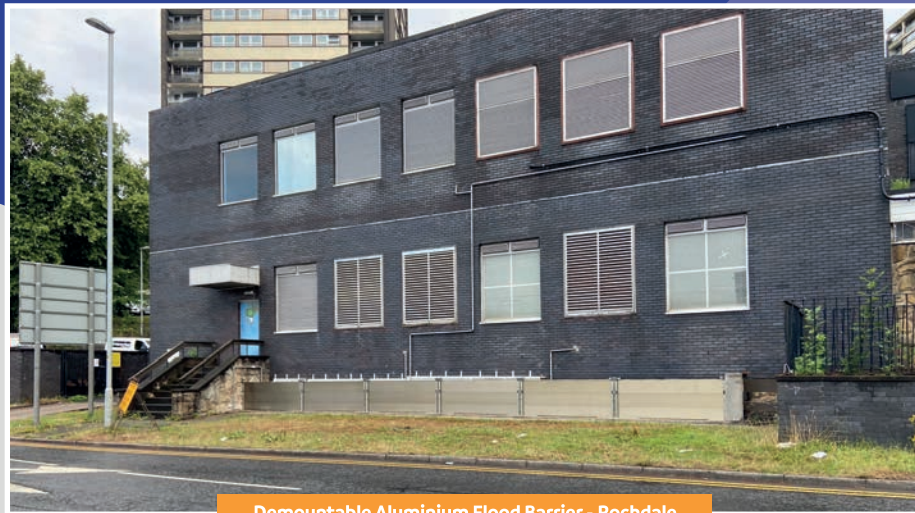
Demountable Aluminium Flood Barrier - Rochdale
