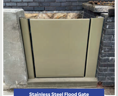
Stainless Steel Flood Gate
