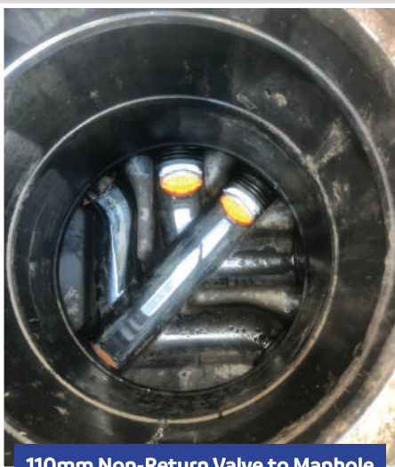
110mm Non-Return Valve to Manhole
