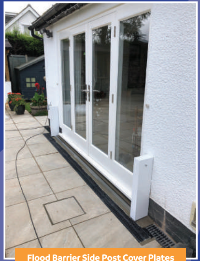
Flood Barrier Side Post Cover Plates
