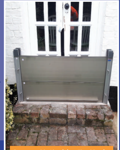
Demountable Aluminium Flood Barrier
